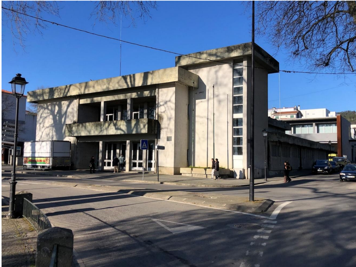
FIGURE 1. FIRE BRIGADE STATION IN ALIJÓ, 2023
